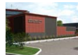
Construction nears completion on radiation centre
